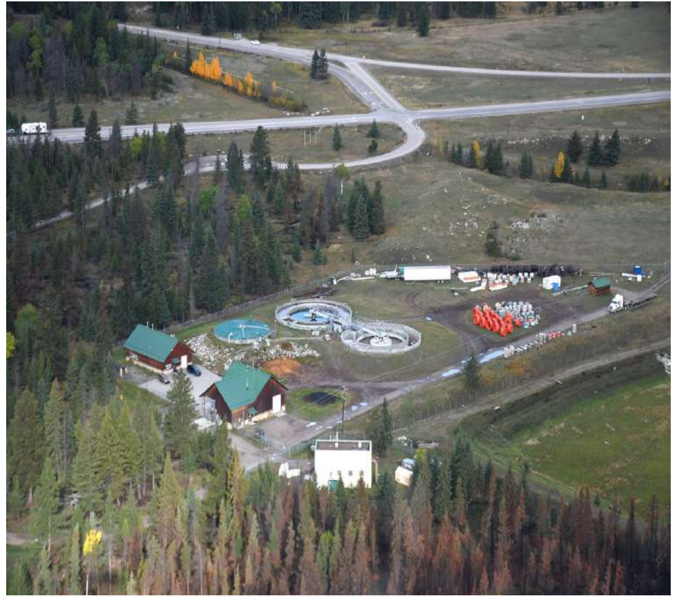
An aerial view of the Jasper Wastewater Treatment Plant. /PETER SHOKEIR, LOCAL JOURNALISM INITIATIVE REPORTER
