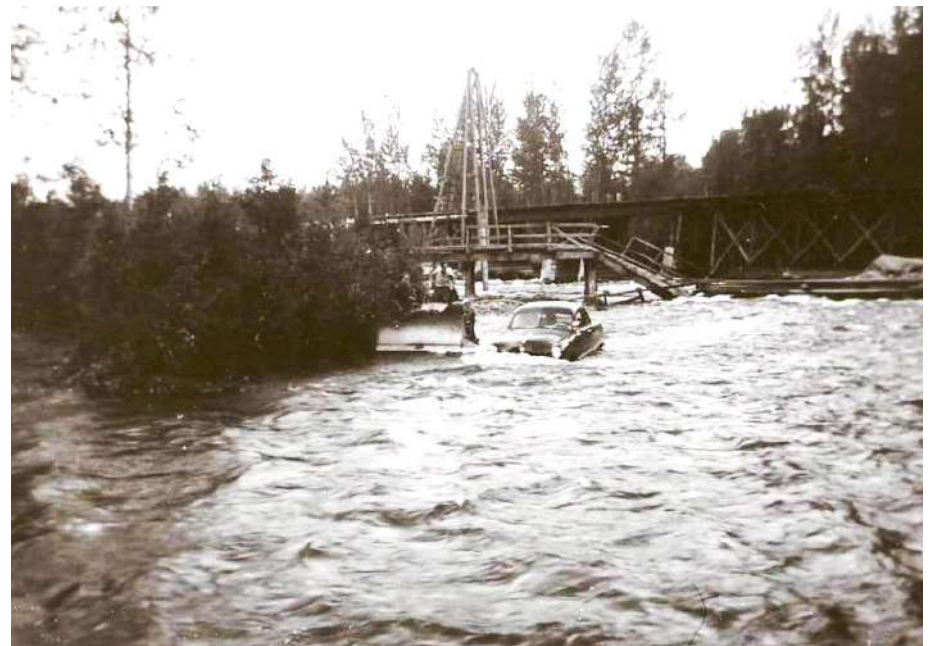
1953 Swift Creek bridge washout. /LLOYD JECK
